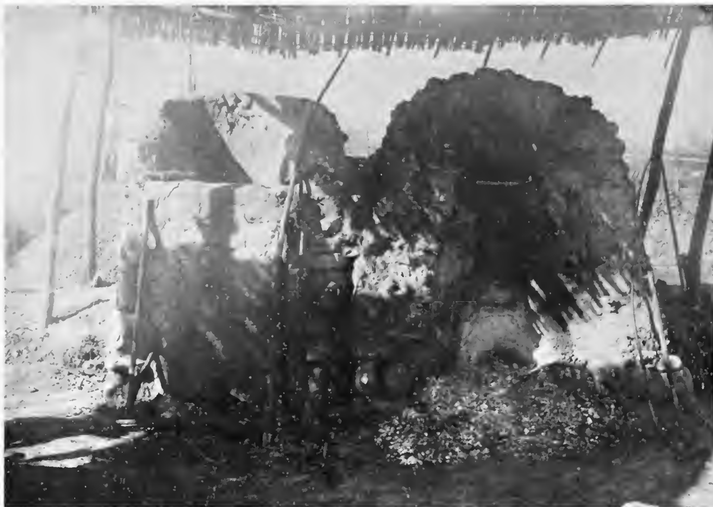
FIG. 2. FRONT VIEW OF LEAD BLAST FURNACES IN THE MING-KUAN.
