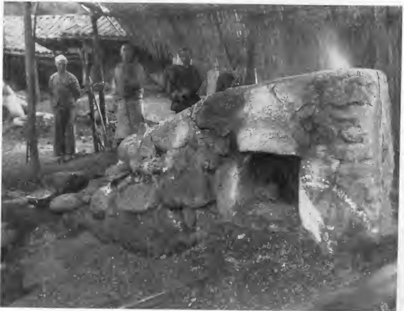
FIG. 2. SIDE VIEW OF THE LOW IRON BLAST FURNACE OF THE TIEN-TAUNG KUAN.
