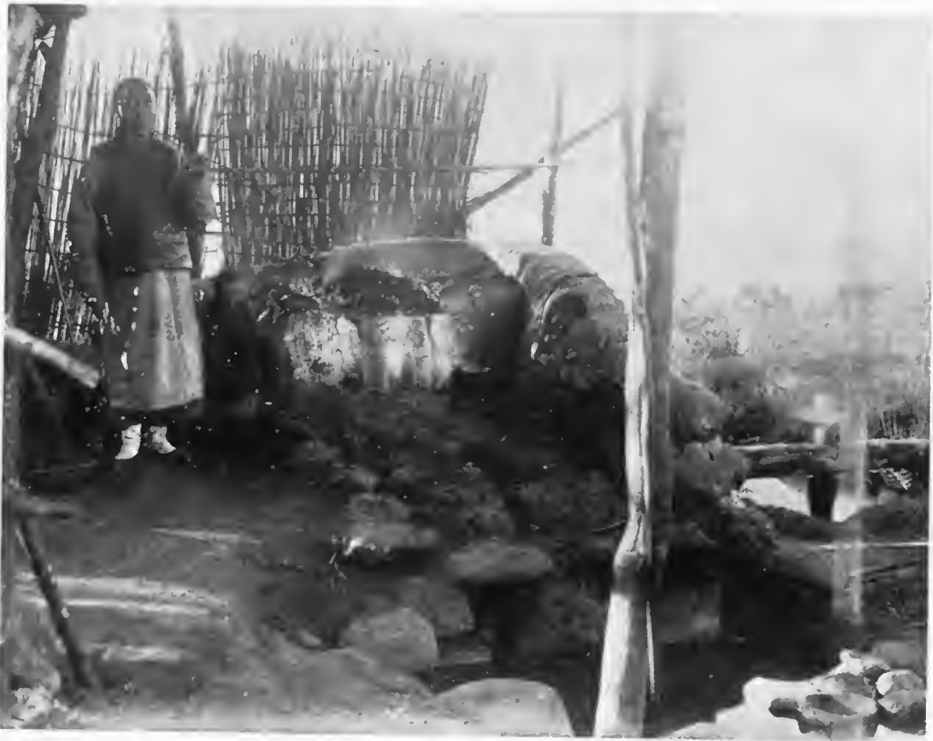
FIG. 1. SMALL IRON BLAST FURNACE IN THE TIEN-TAUNG KUAN, FRONT VIEW.
