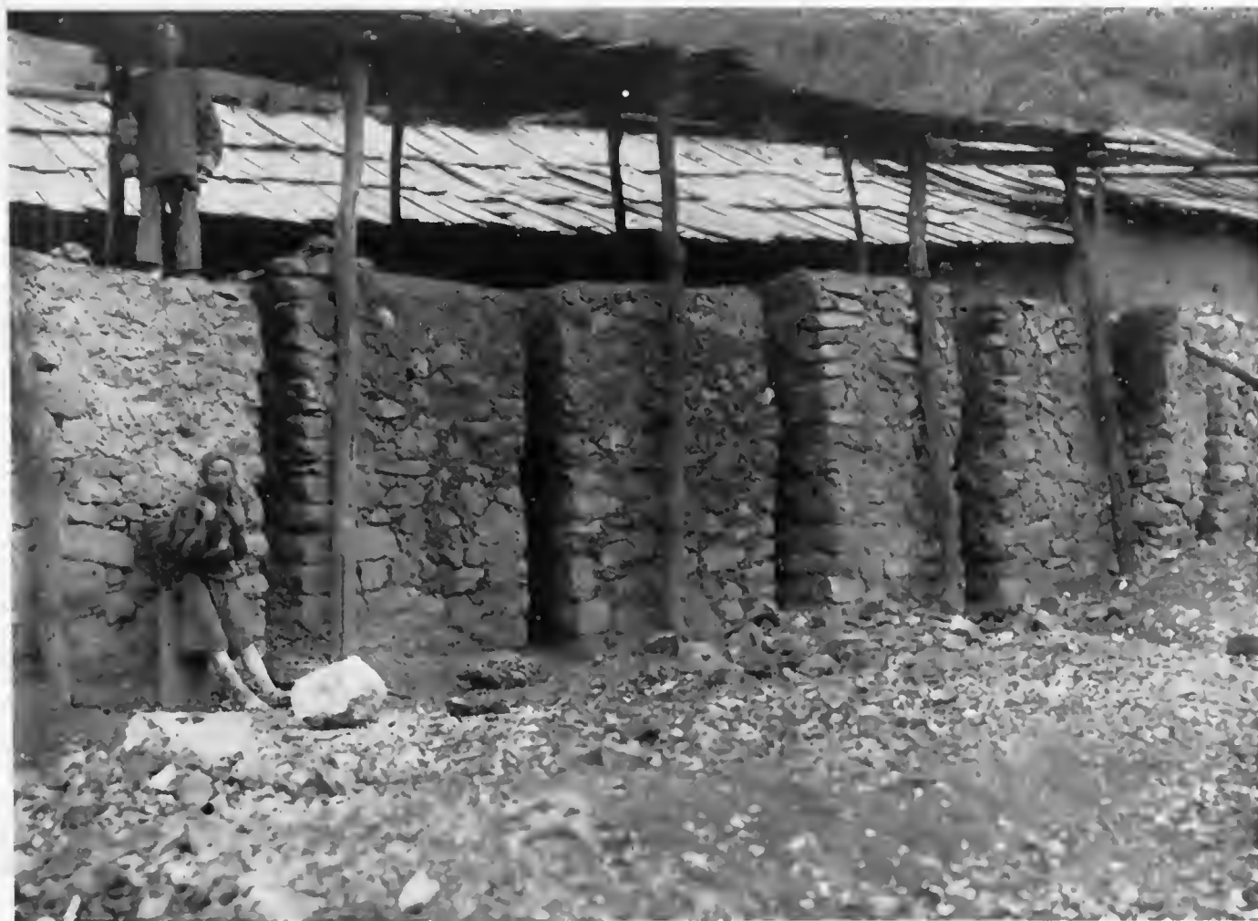
FIG. 1. KILNS FOR CALCINING COPPER ORES, PO-P'ING-CH'ANG.
